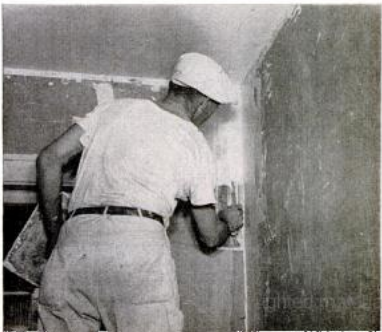
Finish coat is applied to break in room corner, below. Ready-mixed plaster may be decorated as soon as dry—in most cases, two days after application
